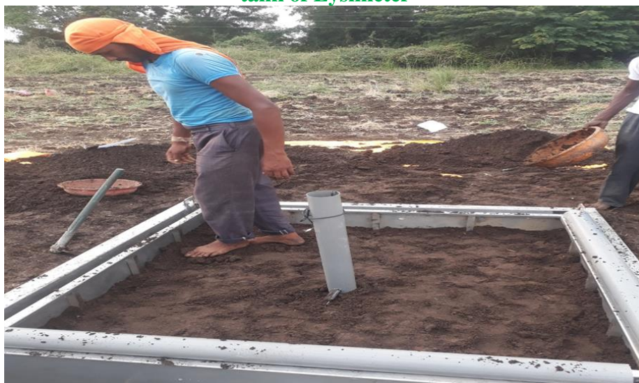
Plate 9. Completion of Soil filling in the inner tank of Lysimeter
