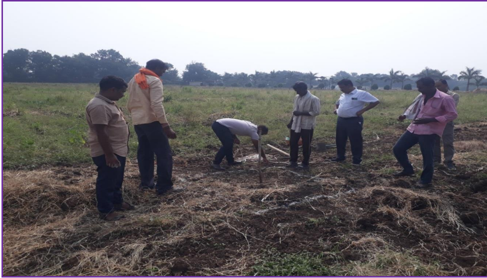
Plate 1. Layout of digging site
