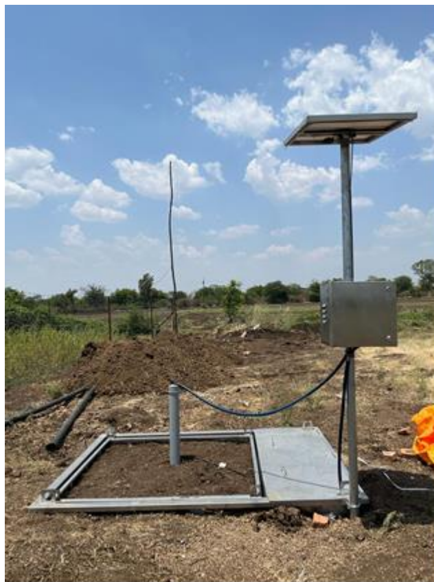
Plate 11. Saturated Lysimeter after successful installation and calibration
