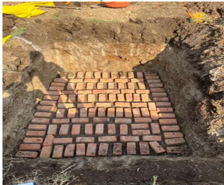
Plate 5. Bricks foundation below Lysimeter as levelled platform
