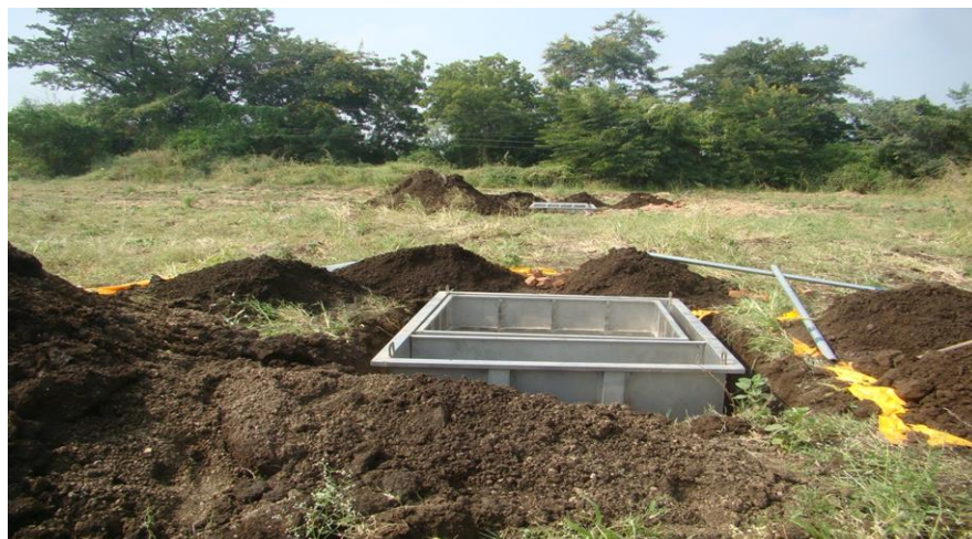
Plate 6. Lysimeter placed on the foundation in pit
